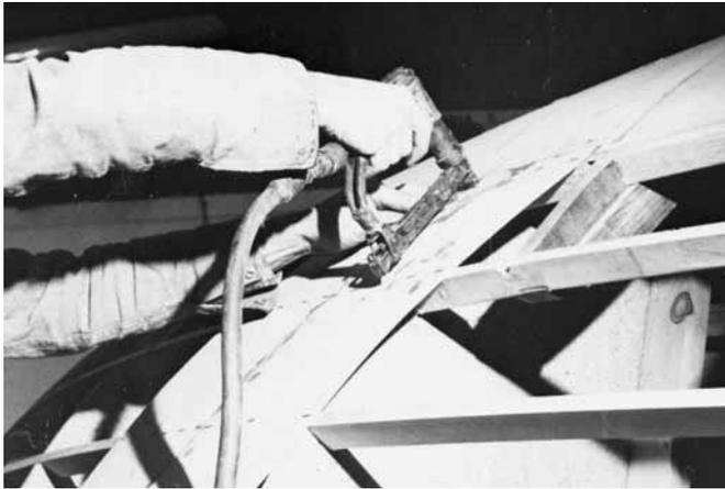
**Figure 22-14** Stapling the first layer of planking to the topsides. Note the laminated curved frame and blocking in the upper right as well as limber holes cut in stringers next to blocking.
