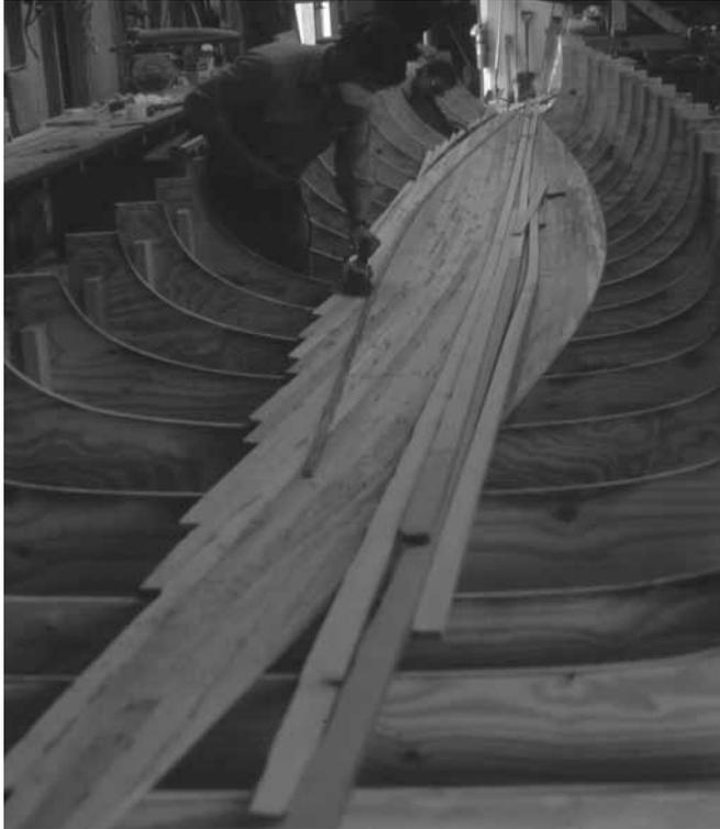
**Figure 23-14** Planking being installed on a mold for the hull of the Formula 40 trimaran *Adrenalin*. The hull was built in left and right female molds rather than the typical male hull and deck molds.
