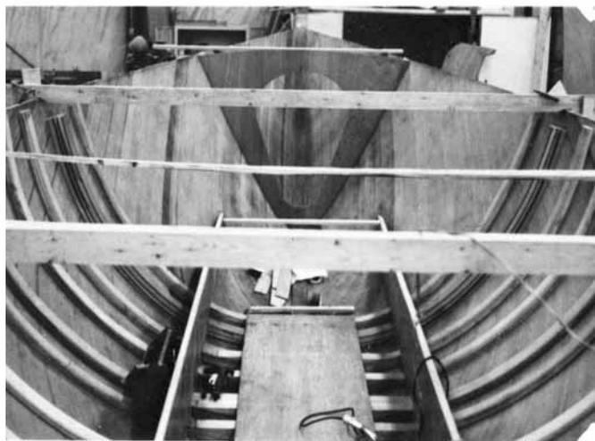
**Figure 11-8** Laminated frames fit to a hull.
