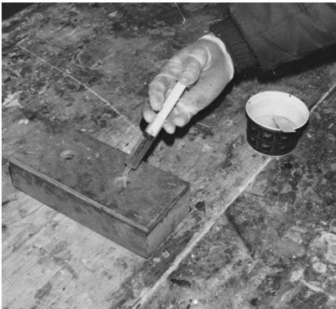
**Figure 14-10** Use a syringe to fill oversized holes.
