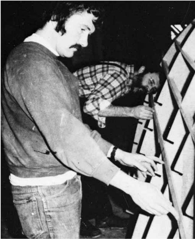
**Figure 22-7** Fairing the molds on a stringer-frame set-up.
