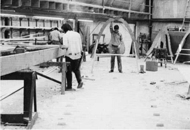
**Figure 18-4** Setting up the first frame.
