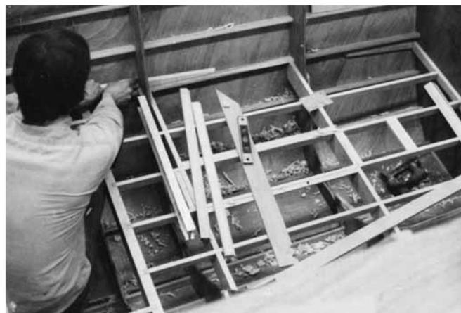
**Figure 26-18** Installing cabin sole framework in *Rogue Wave*. The structure supports the hull skin as well as the cabin sole.
