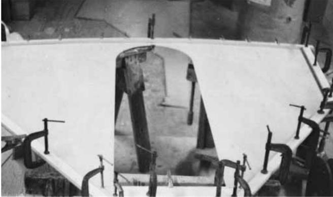
**Figure 17-7** Bonding cheek pieces to a permanent bulkhead.
