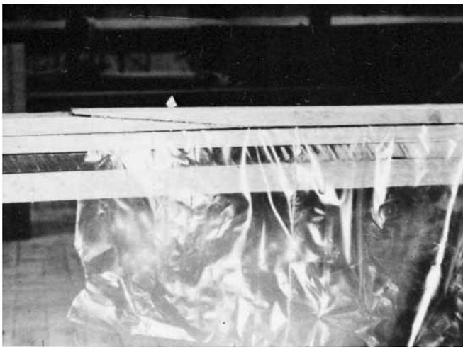
**Figure 12-5** Plastic sheeting woven back and forth between stringers contains the excess epoxy runout and prevents bonding of the stringers to each other. When placing this plastic sheet, avoid pinching the plastic in any of the scarf joints.
