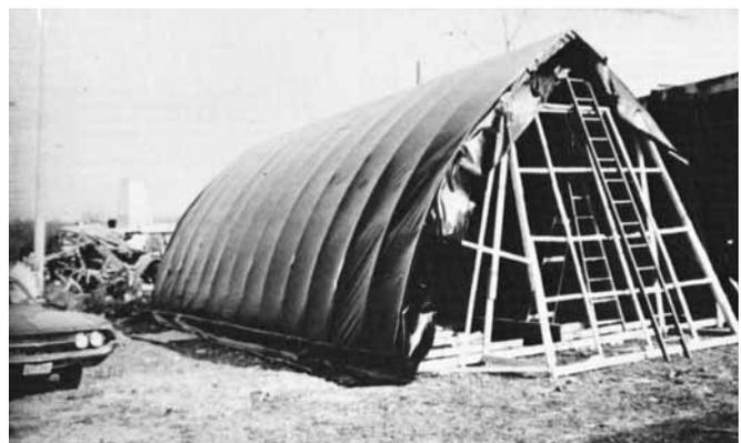
**Figure 8-17** Plastic covering stretched over framework.
