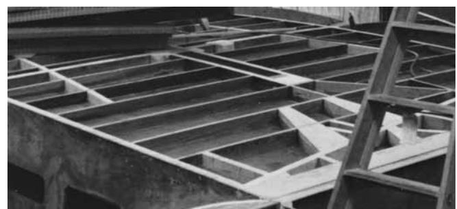
**Figure 27-23** Sawn Sitka spruce blocking is bonded to core deck at all structural frames and planed flush with the deck profile. Note the strip of blocking for adjustable sail leads to the left.
