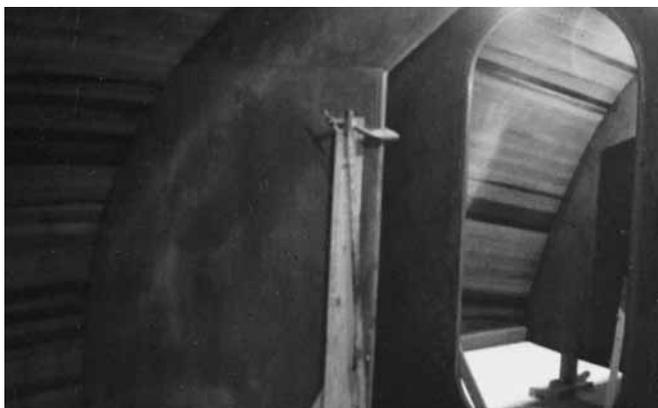
**Figure 23-10** The 42' hull with the temporary mold removed. The hull is supported by permanent bulkheads installed during set-up. Note the clean interior in which work can progress while exterior finishing is completed.
