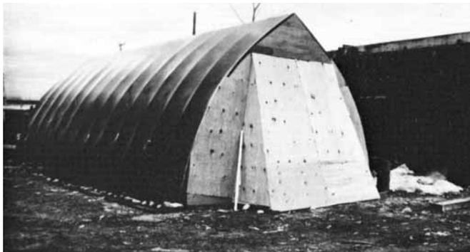
**Figure 8-18** Shelter completed. Plywood walls were used at both ends to give the structure extra rigidity.
