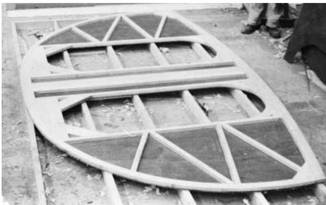
**Figure 26-12** A major structural bulkhead for *Golden Dazy* is constructed with a framework sandwiched between two  $\frac{1}{2}$ " (12mm) thick panels of utility plywood.
