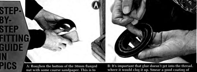
give a good "key" for the adhesive to ensure it won't vibrate loose when fixed to the boat hull. Vaseline right around the threads - make sure it doesn't get on the bottom of the flange.
